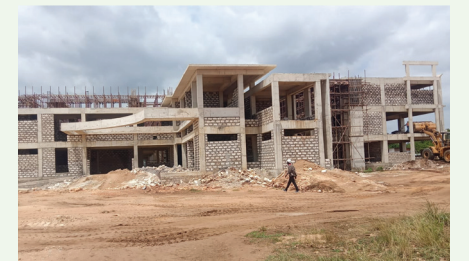
Ongoing construction of KCNP's Maritime Centre in Kombani, Kwale County.
